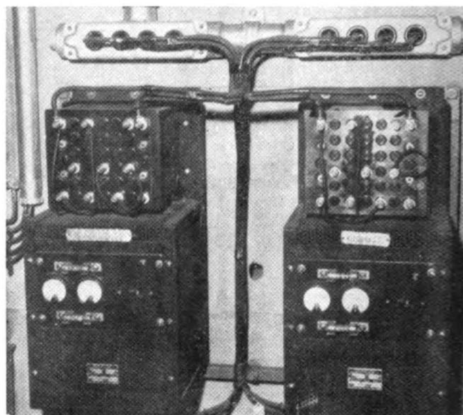
These rectifiers supply 16-volt d.c. for control circuits of signals and switches
