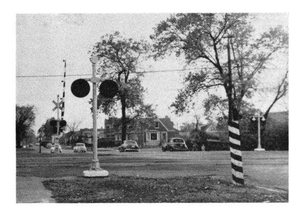
At the left in this picture is one of the new pedestrian signals, directed along sidewalk
