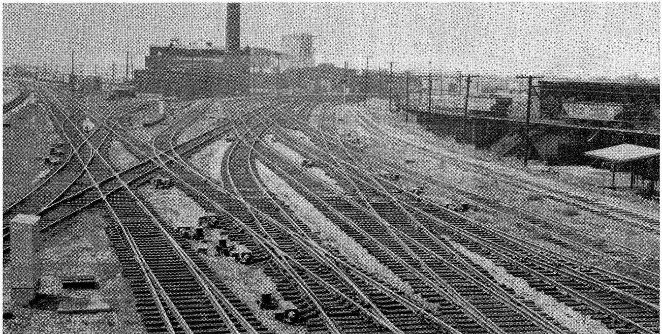
Seven non-conflicting routes can be lined up through these switches and slips
