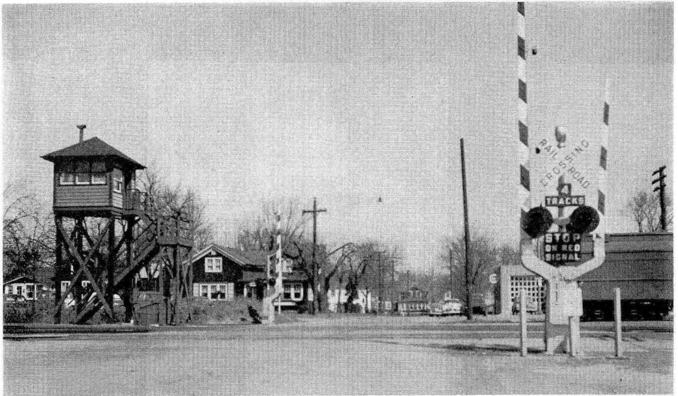
One mechanism operates street arm and sidewalk arm
