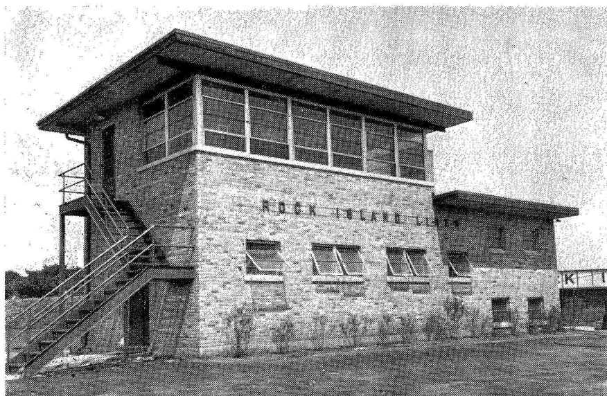
The new tower is of concrete and brick fireproof construction
