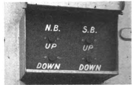
Gates and flashers at Washington ave., Racine (left) can be controlled manually (above) when switching moves are made
