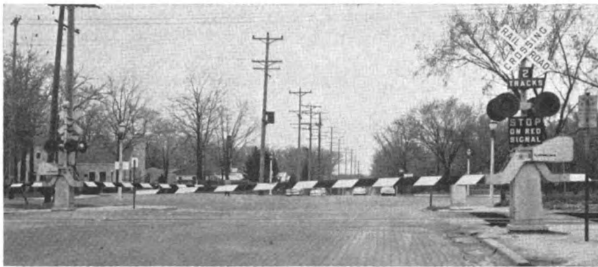
Gates and flashers at Washington ave., Racine (left) can be controlled manually (above) when switching moves are made
