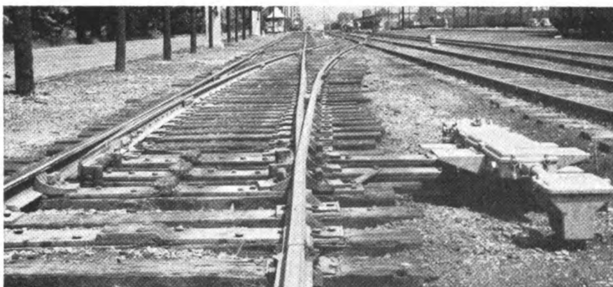
Insulated gauge plates extend under 110-volt d.c. switch machines
