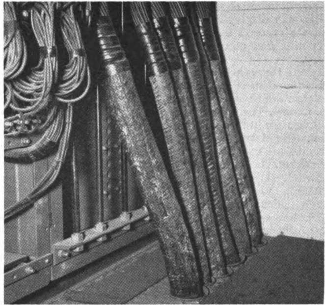
All wiring enters the tower in underground cable
