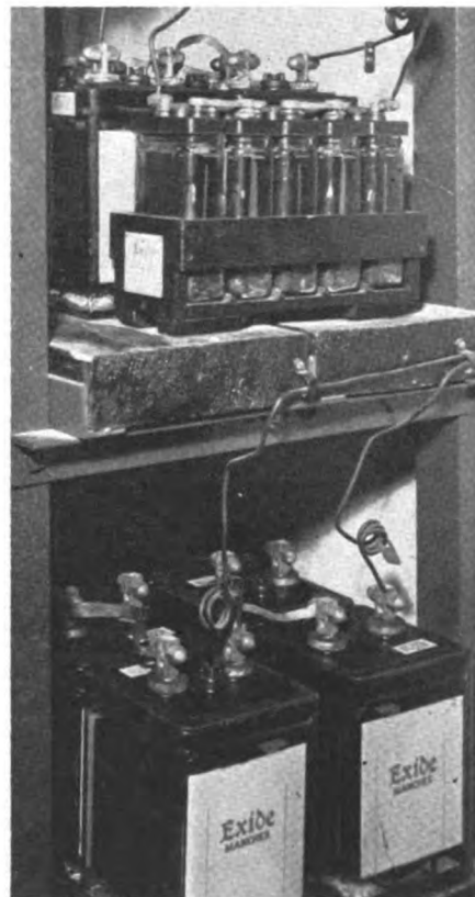
Batteries in open racks
