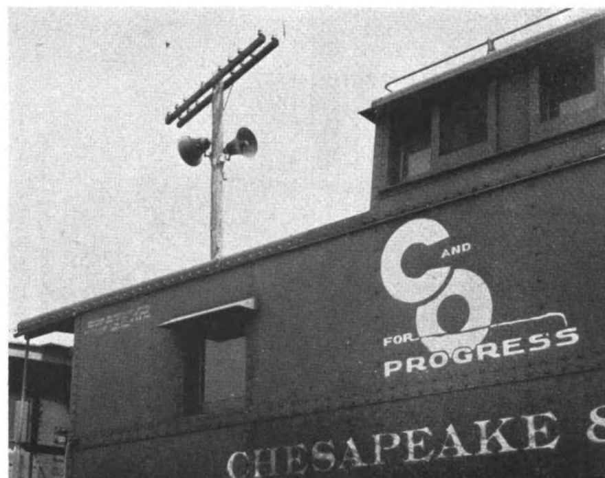
Paging speakers mounted high above ground to provide coverage over several tracks
