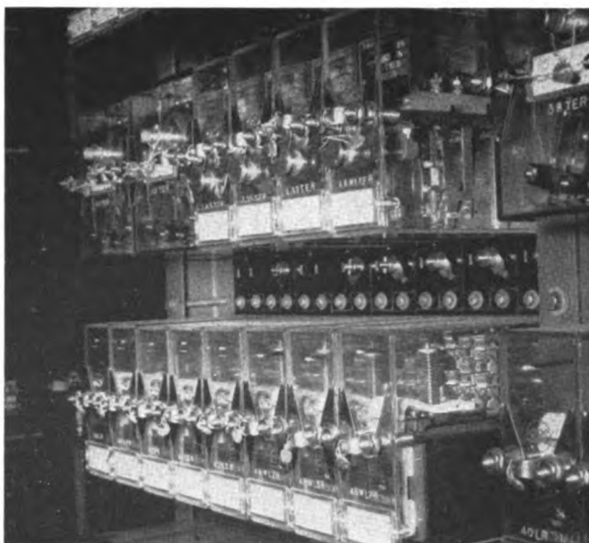
Plug-in relays used extensively at instrument housings
