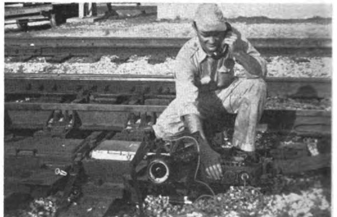
Electric switch machines are equipped with telephone jacks enabling maintainers to talk with interlocking operator
