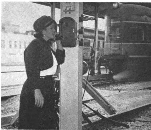
Train starter telephones to interlocking tower to inform leverman that a passenger train is ready to depart
