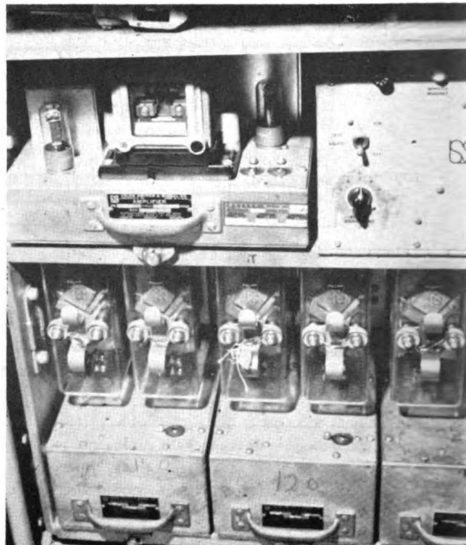
Cab signal equipment is rack-mounted in nose of locomotive
