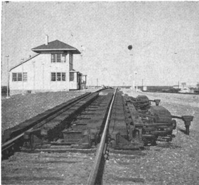
After passing yard office, cars go through this master retarder . . .
