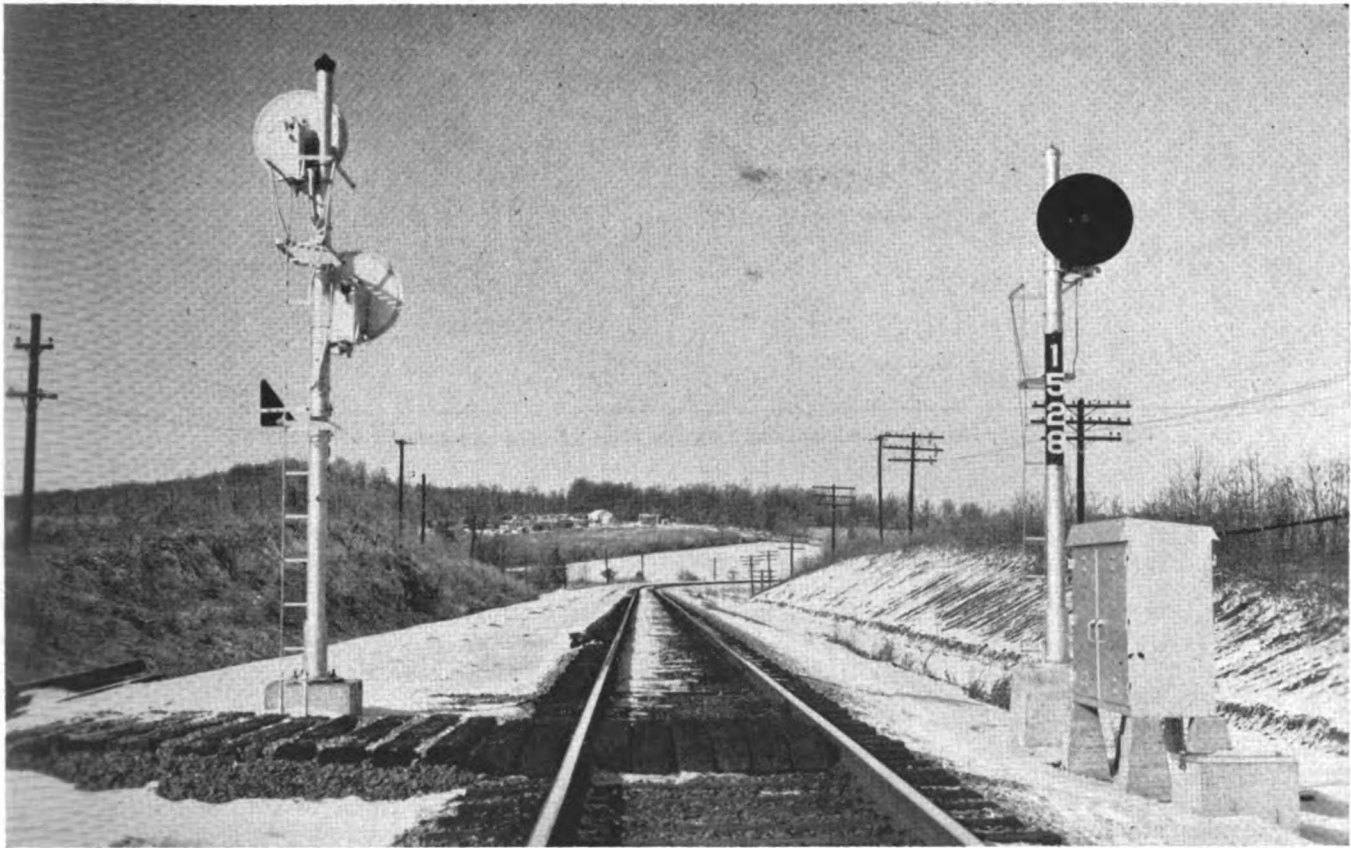
Intermediate location—approach signal (left) in advance of double track may display "Approach Limited"
