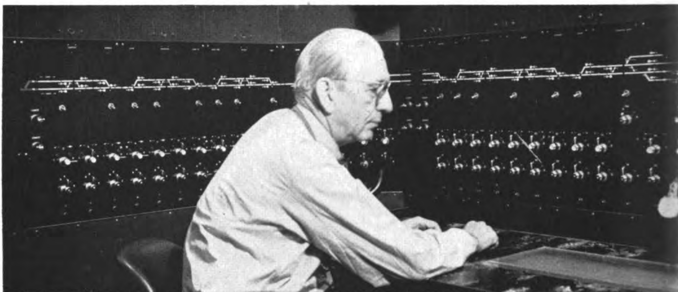
The centralized traffic control machine is in the dispatcher's office at Somerset
