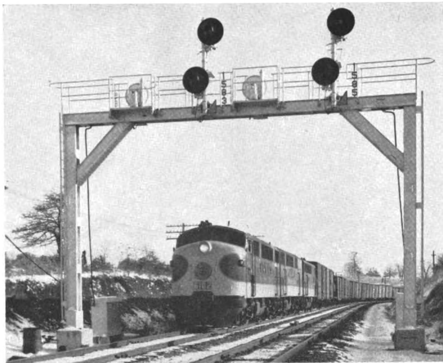
Intermediate location—two-unit signals are in advance of a double crossover
