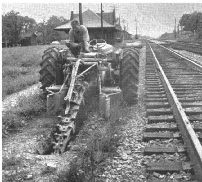
TRENCHER can dig a trench 42 in. deep for underground cable
