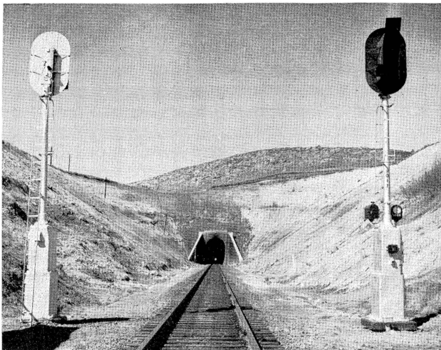
EAST END ALTAMONT TUNNEL looking west toward Ogden. Switch-key controller and indicator lamp are mounted on end of signal case, below motor car indicators. When controller operated by switch key, home signals at each end of tunnel will display flashing-red aspects. First signals in approach will display yellow, second signals in approach will display flashing-yellow and third signal in approach will be green
